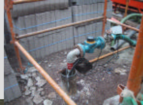
Wellhead under construction
